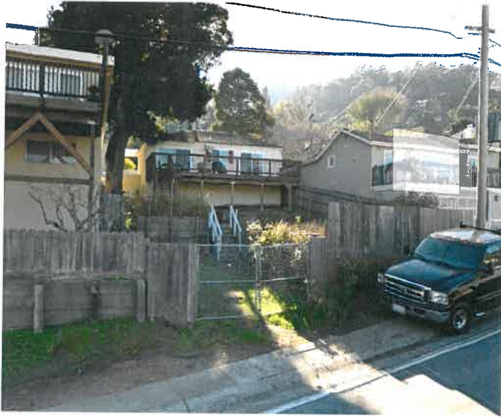
119 San Benito Road Existing structure, rear elevation (from Visitacion Ave)
