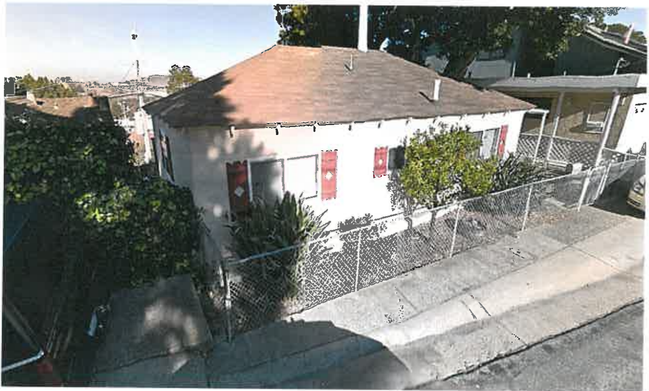
Existing structure, front elevation (San Benito Rd)
